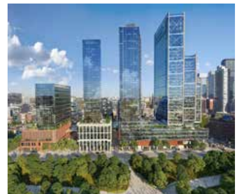
In Toronto, BDP has designed a three-level retail podium for RioCan at The Well – a large mixed-use commercial development, currently under construction. Photo: © BDP
