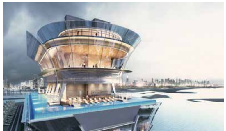
The Palm Tower's rooftop pool, and the restaurant and viewing deck podium being built above it on floors 51 and 52. Photo: © Nakheel
